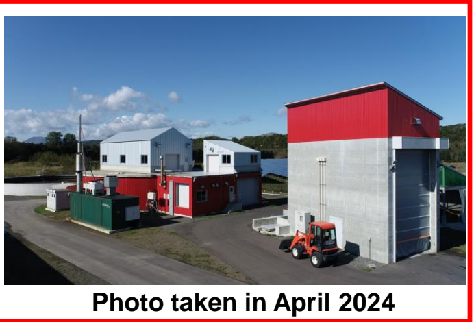
Hokko bio-gas plant
