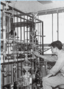
Large-scale falling-film vacuum distillation equipment
